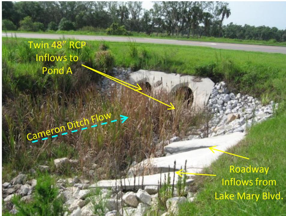
Figure 2-3. Photograph of the Culvert Structures on the North Side of East Lake Mary Blvd.
