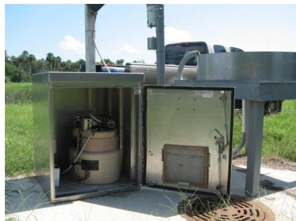
b. Autosampler inside insulated equipment shelter
